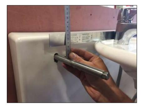
Turn washbasin in against the cover. Place if possible a spirit level onto washbasin. For fitting of fixation of Dock-in to be fastened in correct height loosen fittings a little & adjust them to leave approx. 33mm between fittings & spirit level. Afterwards fasten fittings thoroughly with a spanner.
